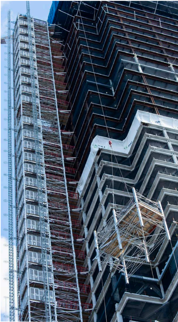
Common Platform pod being picked by crane to the setback floor.
